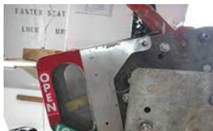
Inadequate re-setting of on-load release gear
