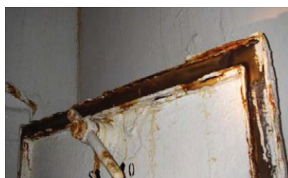
Corroded packing
